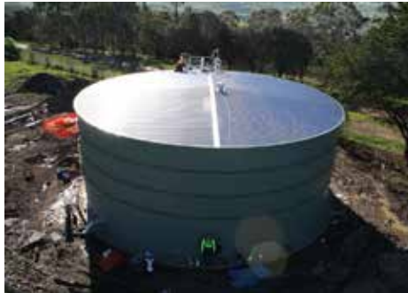
Coleraine 950kl clearwater storage tank with reinforced Aeon Liner and stainless steel roof
