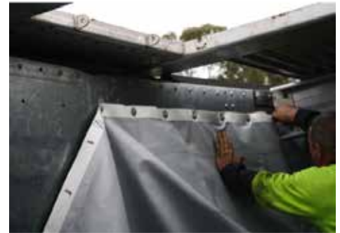
PVC liner installation
