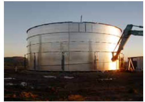
Mansfield 1000kl clearwater storage tank with reinforced Aeon Liner, shown with bare galvanised finish
