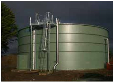
Mansfield 1000kl clearwater storage tank with reinforced Aeon Liner, shown with bare galvanised finish
