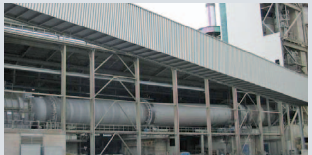
Cement industry – rotary kiln feed
