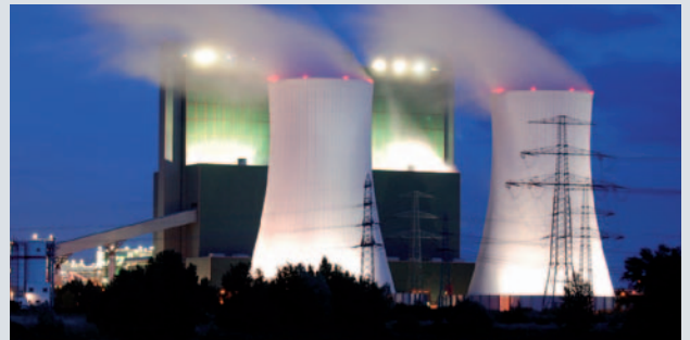
Energy/power plants – flue gas desulphurization
