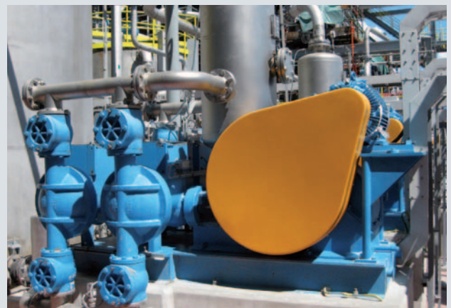
ABEL HMQ with duplex stainless steel wet ends for autoclave feed
