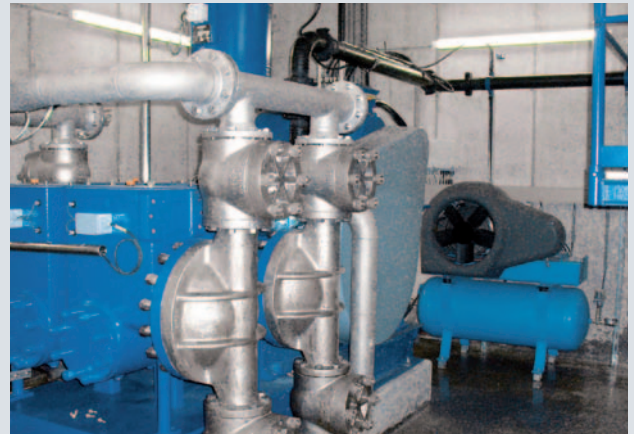
ABEL HMQ with stainless steel wet ends for transporting brine slurry
