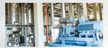
Ammonia (Refrigerant R-717) is a very thin liquid that is a gas at ambient temperature and pressure. It is typically kept at elevated pressure to keep it in liquid form. Ammonia is used as the refrigerant in cooling systems.
